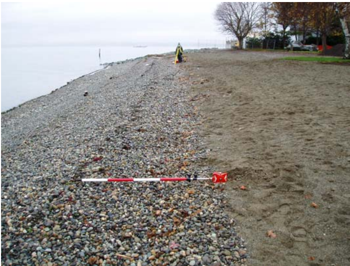
Marine Park, Fairhaven (Bellingham): Pre-project, immediately Post Beach Rehabilitation (early Nov. 2004), and post-storms (Nov. 22, 2004). Removal of fill, rock, and debris and importation of gravel, backshore sand, and 2 rock drift sills. Pre-planting following beach design by Jim Johannessen of Coastal Geologic Services and drift sill & revetment design by Reid Middleton.
