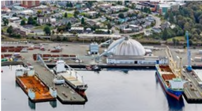
FIGURE 8 – EVERETT SHIP REPAIR
