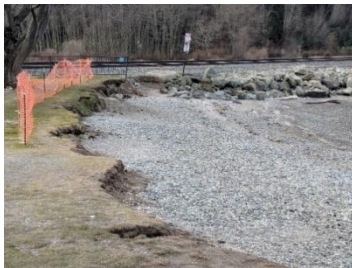
Erosion at Marine Park, 2018
