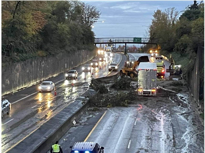
Northbound lanes of I-5 in Bellingham blocked by debris after heavy rains. October 2024, WSDOT
