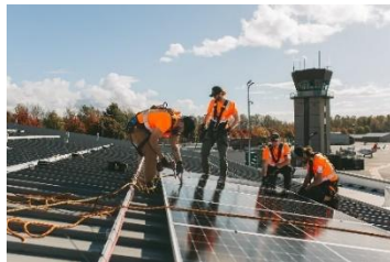
BLI Solar Panel Installation, October 2024
