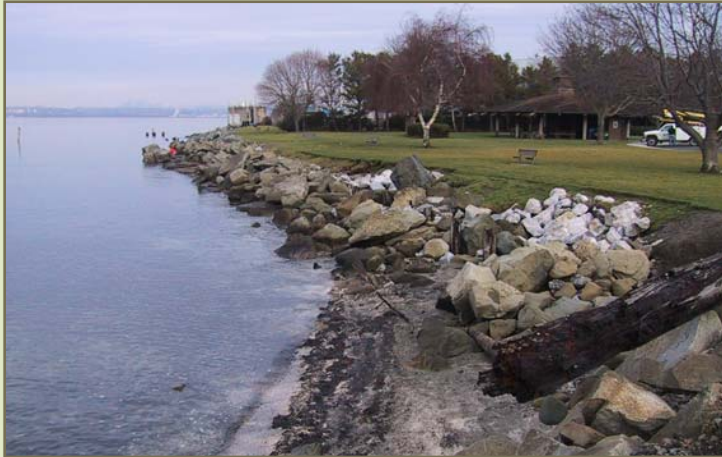
Marine Park, Fairhaven 2004 Beach Rehabilitation Project
