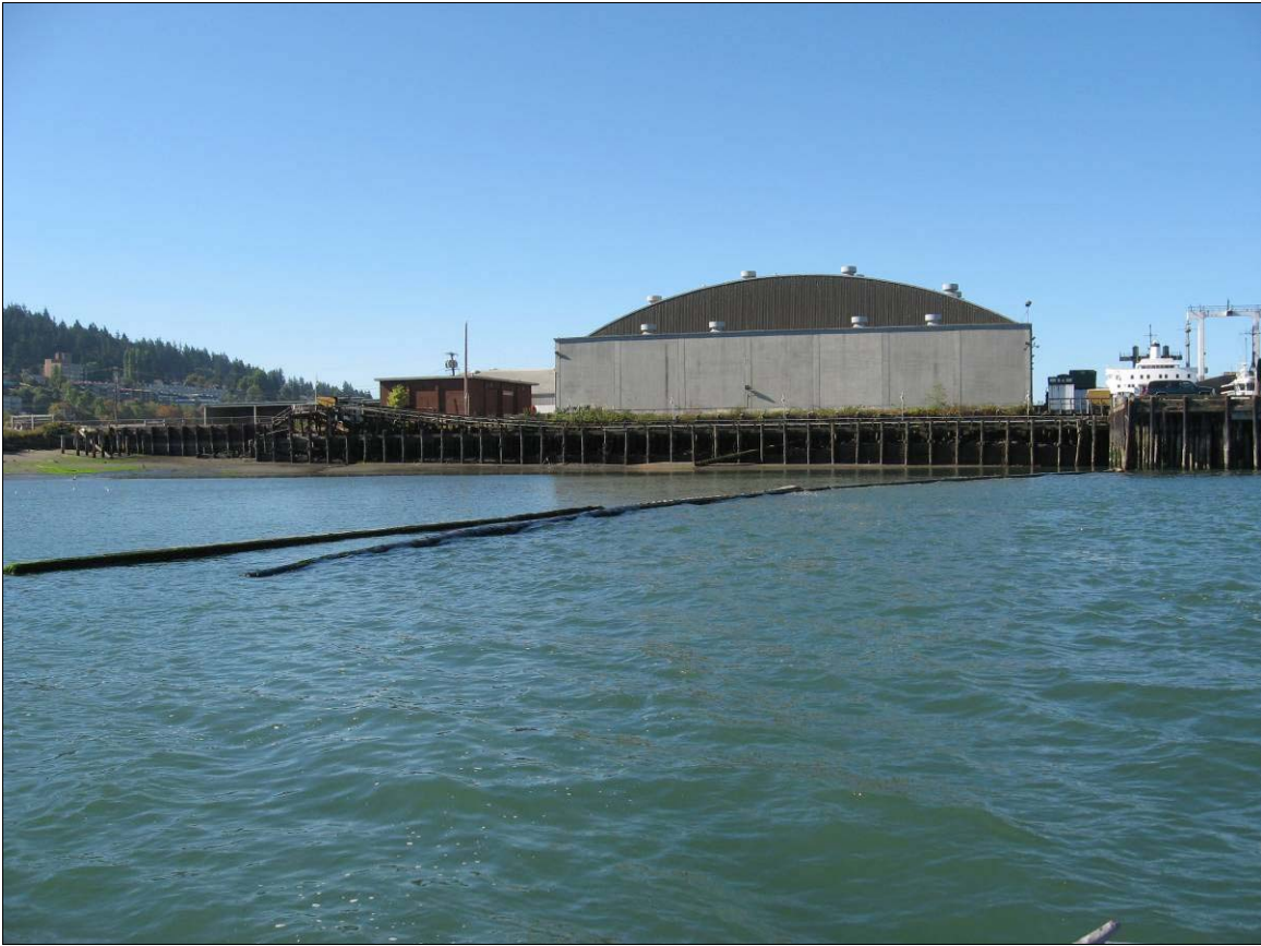
Photograph 9. Pier, bulkhead in western portion of log pond in Areas 8 & 9
