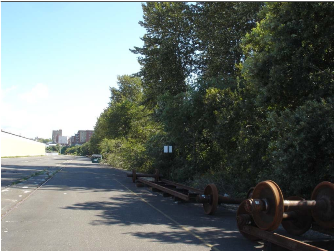
Photograph 8. Pavement, railroad infrastructure in Area 7 adjacent to wetland complex
