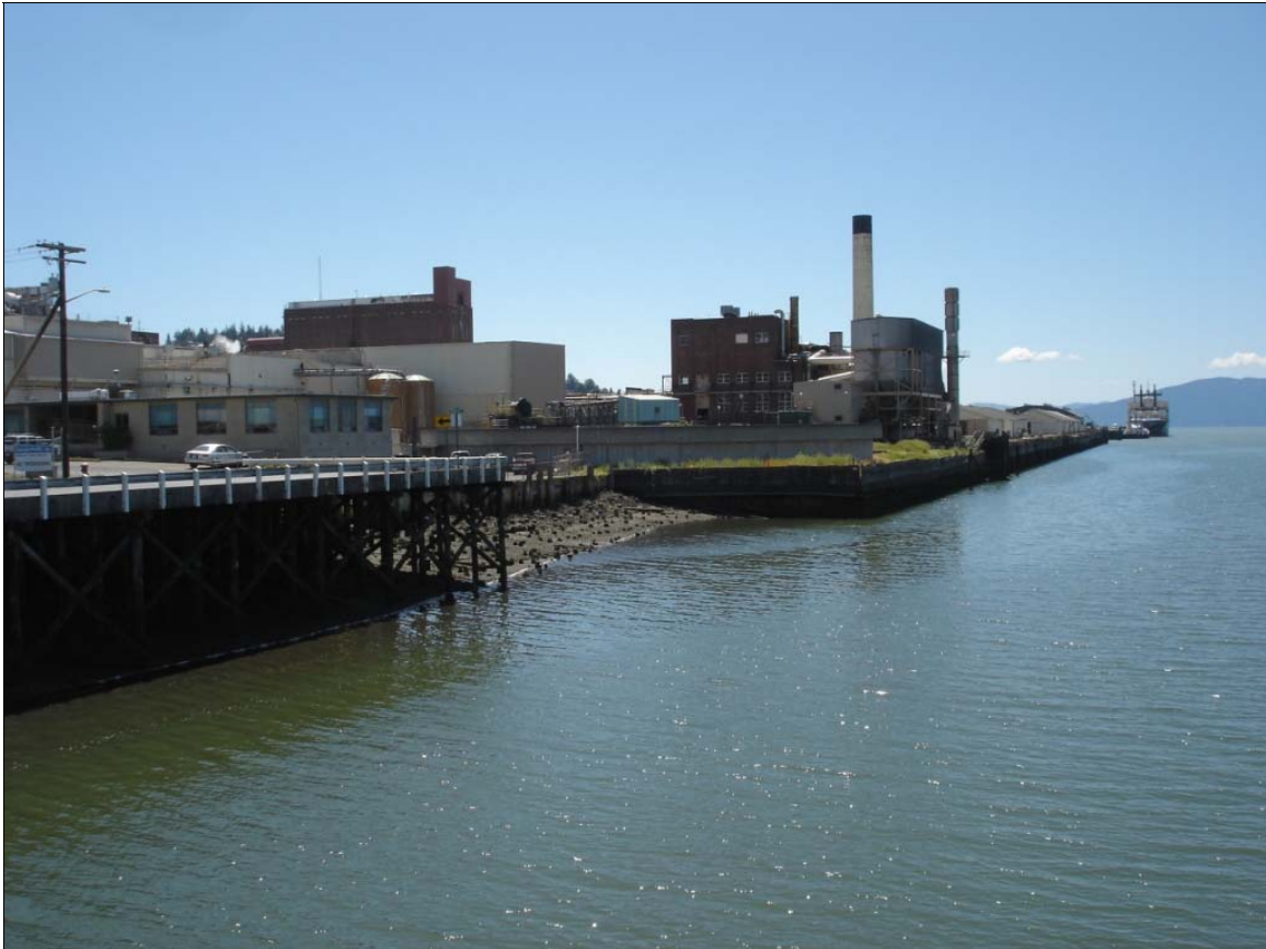
Photograph 5. Pier, bulkhead, cut slope along Areas 2-4 shoreline
