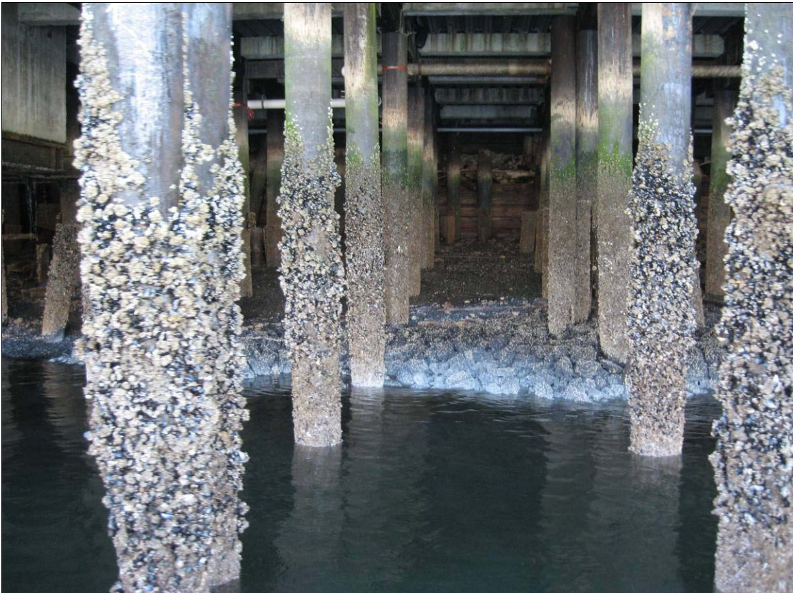
Photograph 6. Typical under-pier conditions in Areas 2-4
