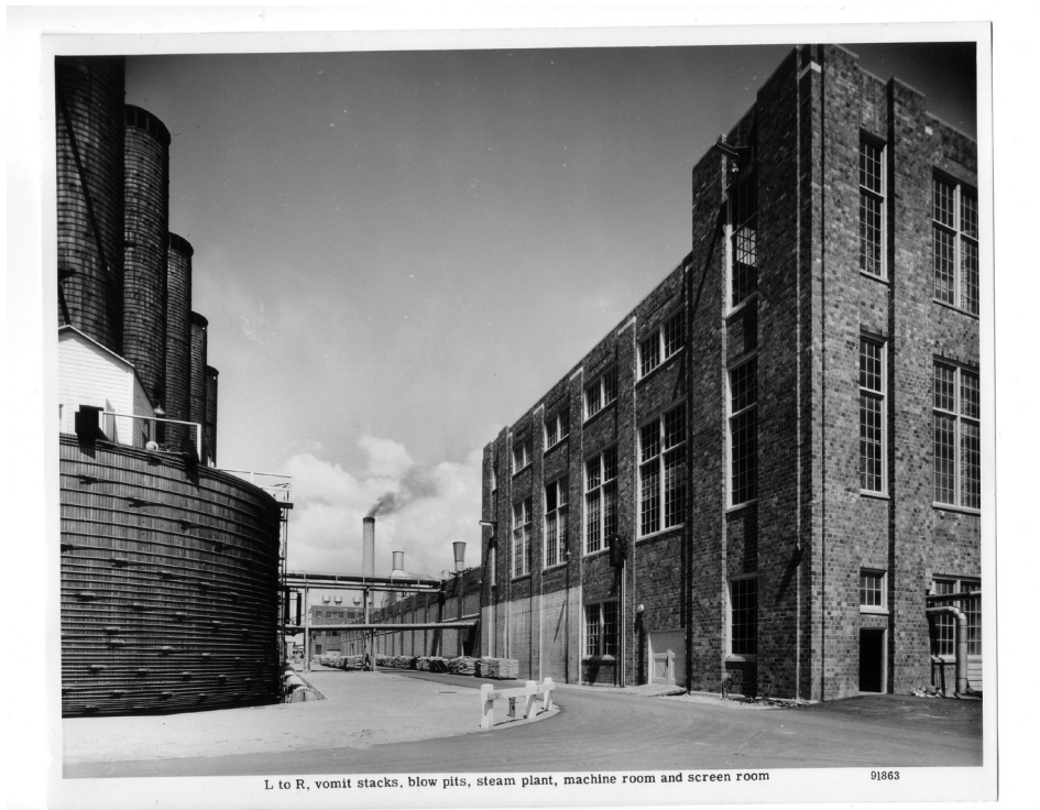
Pulp mill facilities. Source: Georgia Pacific.
