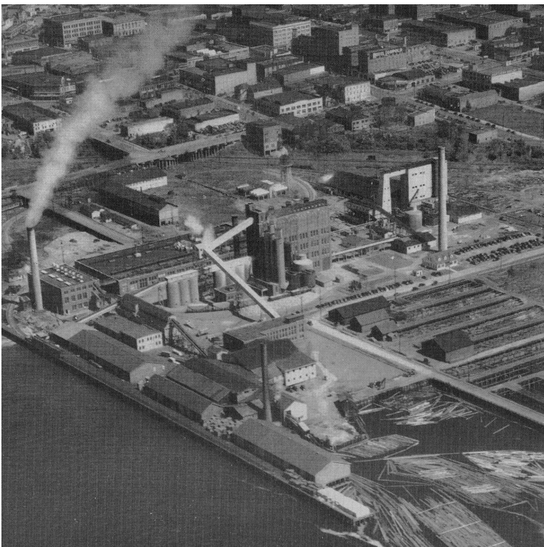
Aerial view of the pulp mill facilities. Source: Georgia Pacific.
