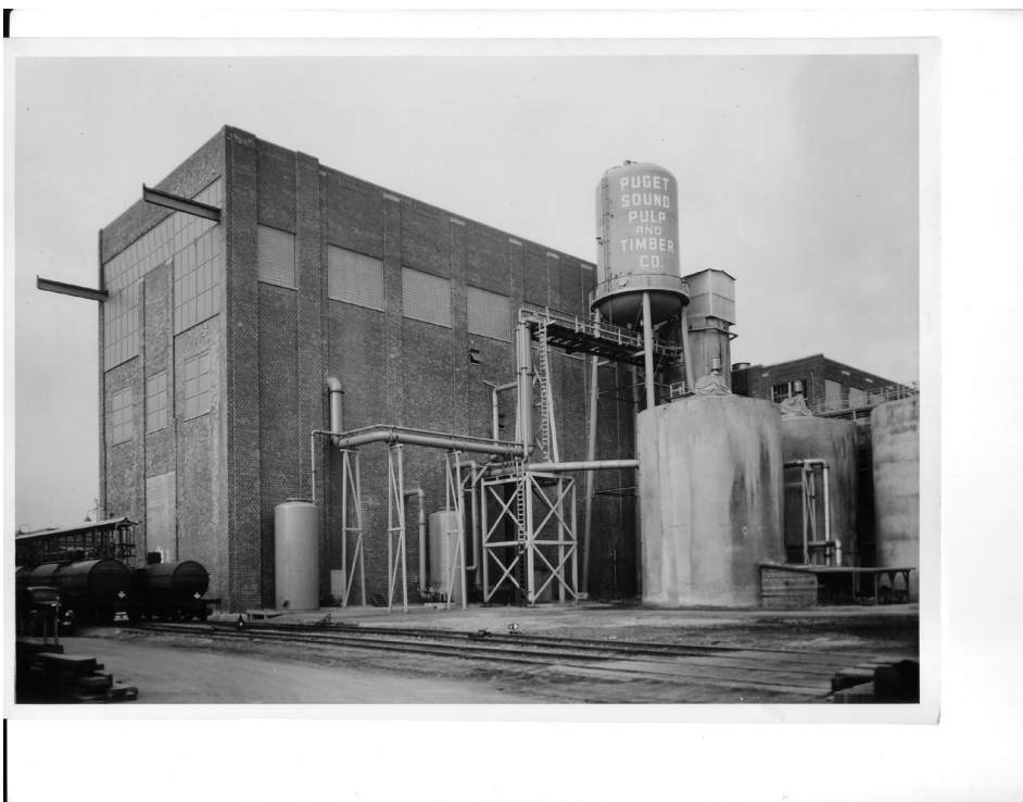
Pulp mill facilities. Source: Georgia Pacific.
