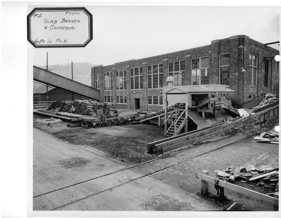
1944 view of pulp mill facilities. Source: Georgia Pacific.
