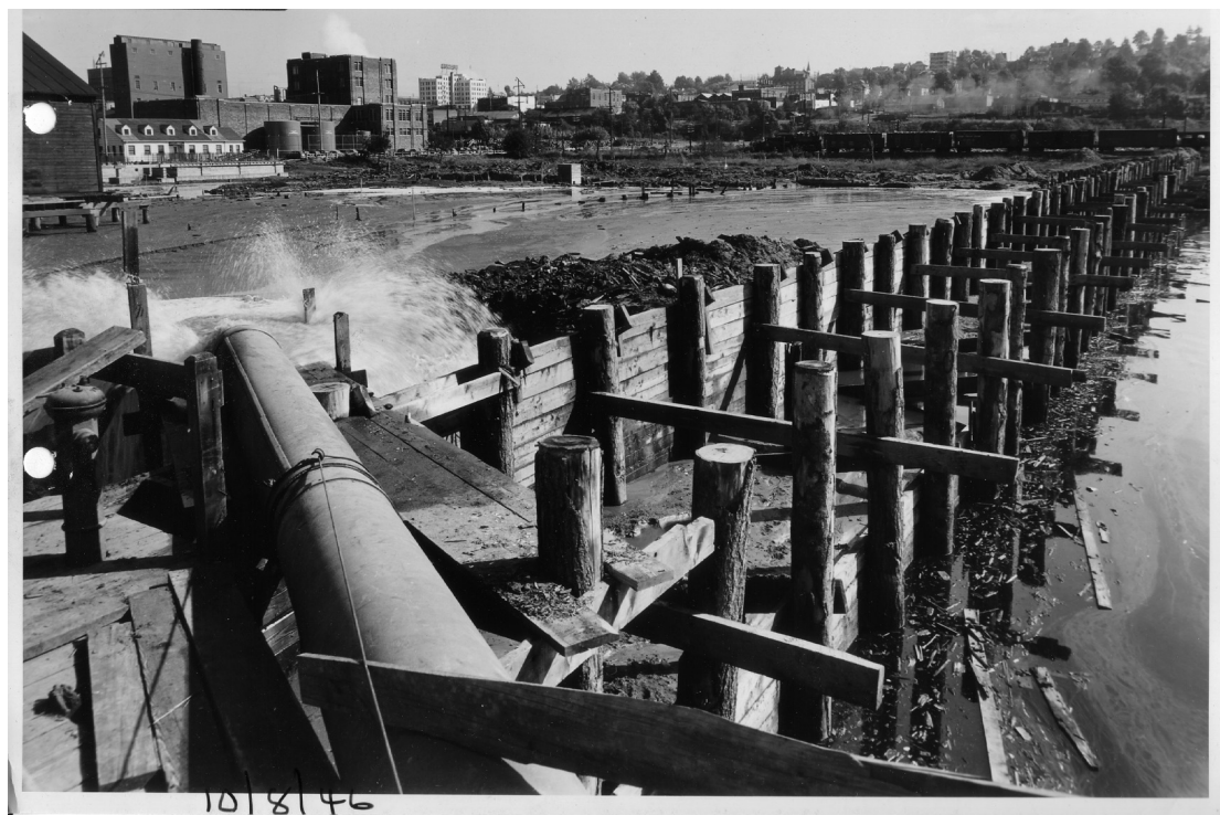
1946 view of bulkhead and fill work. Source: Georgia Pacific.
