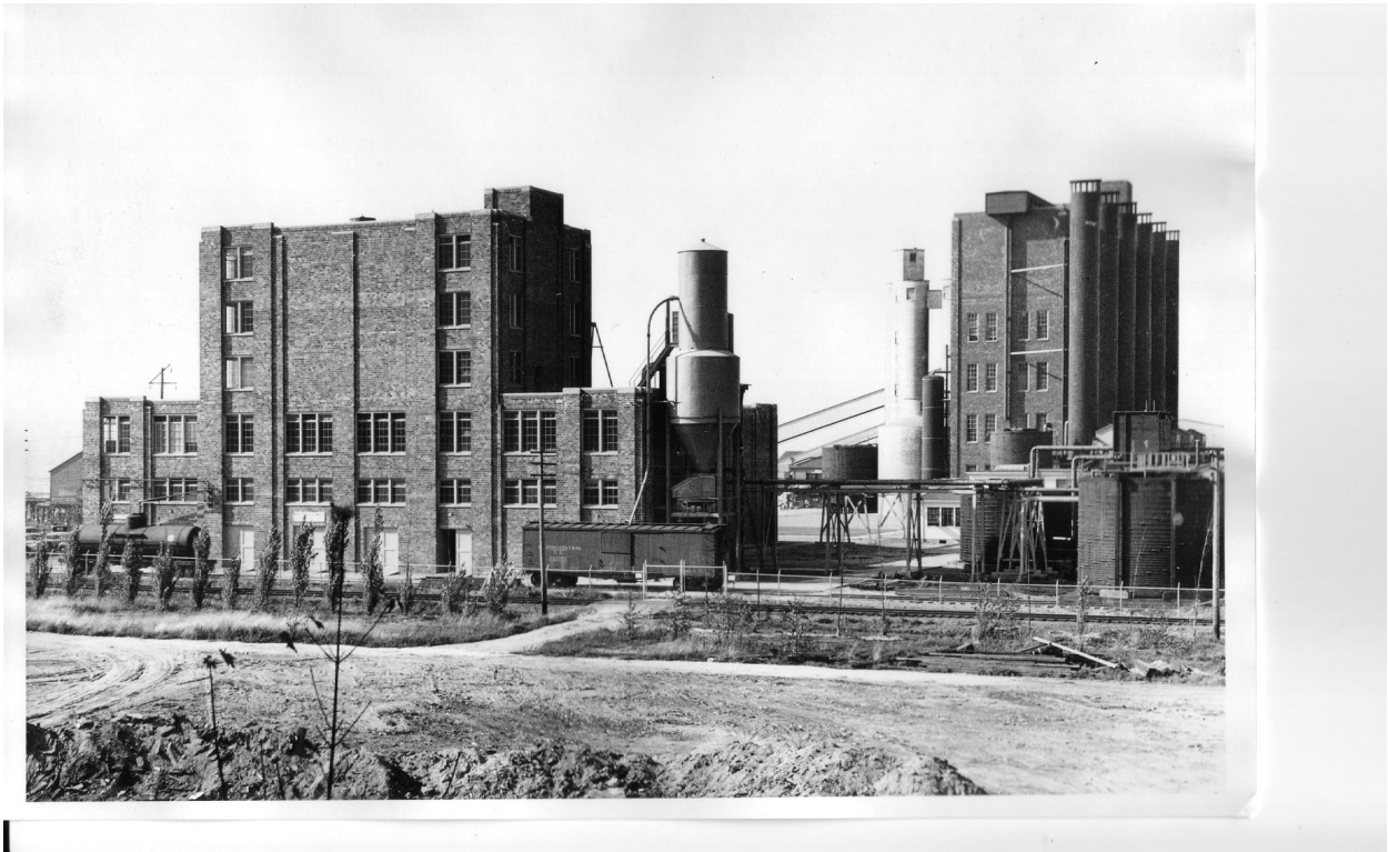
Pulp mill facilities. Source: Georgia Pacific.
