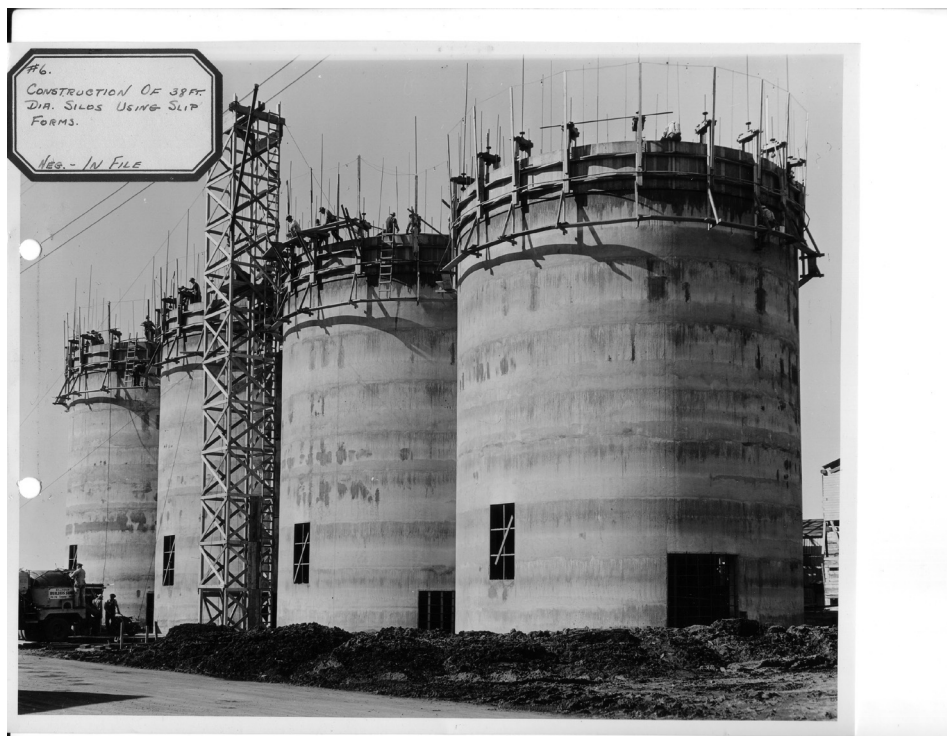
Pulp mill facilities. Source: Georgia Pacific.
