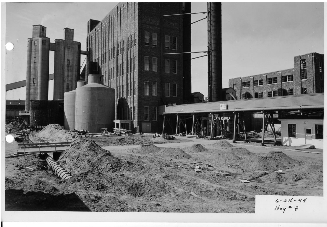
Pulp mill facilities. Source: Georgia Pacific.
