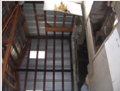
View of East end volume taken 8/29/2006 Photography Neg. No (Roll No./Frame No.): 10 Comments:
