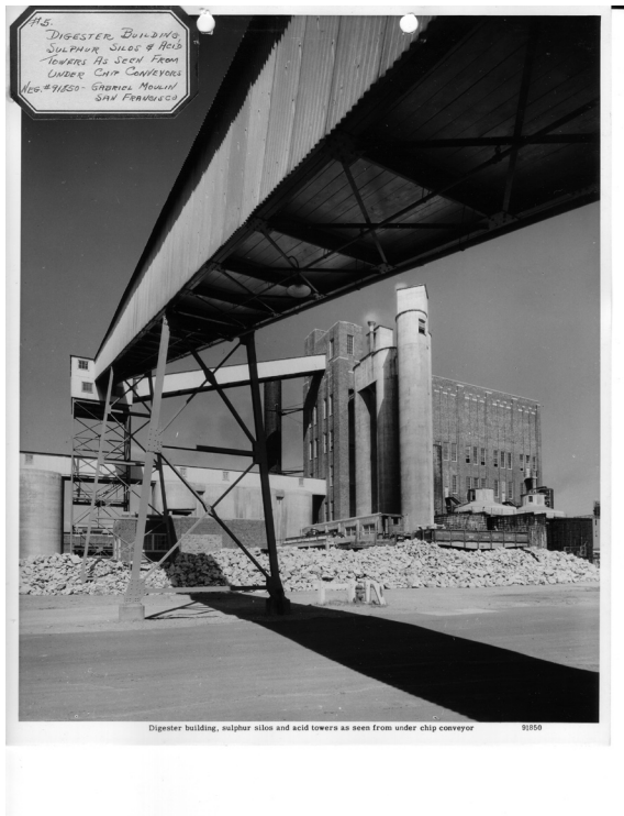
Pulp mill facilities. Source: Georgia Pacific.
