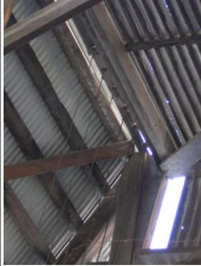
View of Wire and roof detail taken 8/29/2006 Photography Neg. No (Roll No./Frame No.): 12 Comments:
