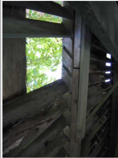
View of louver detail taken 8/29/2006 Photography Neg. No (Roll No./Frame No.): 10 Comments:
