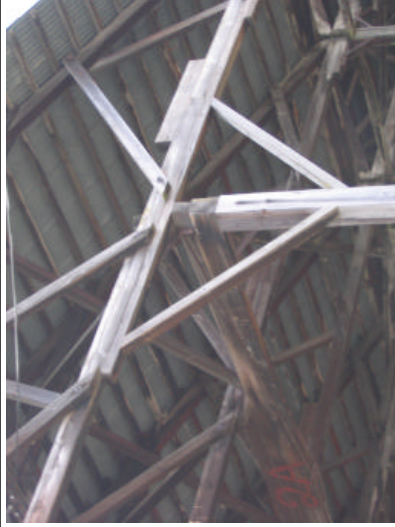
View of framing detail taken 8/29/2006 Photography Neg. No (Roll No./Frame No.): 4 Comments:
