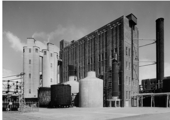
View of the Georgia Pacific Pulp & Tissue Mill facilities. Source: Georgia Pacific.
