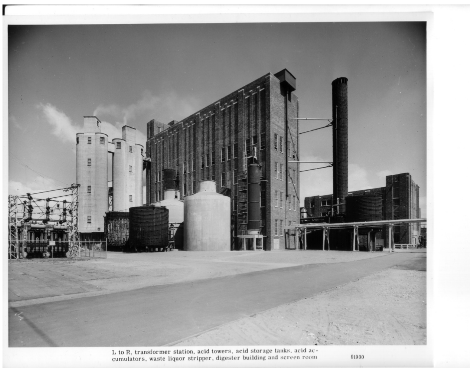
Pulp mill facilities. Source: Georgia Pacific.
