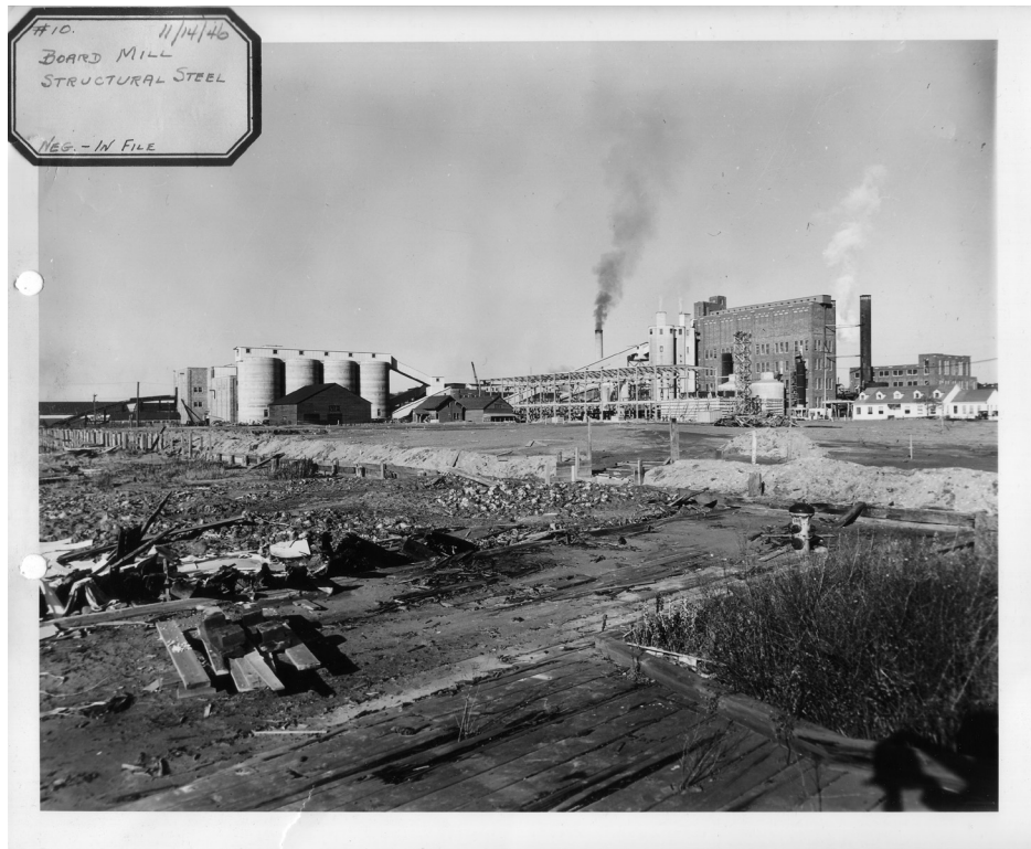
1946 view of construction of pulp mill facilities. Source: Georgia Pacific.
