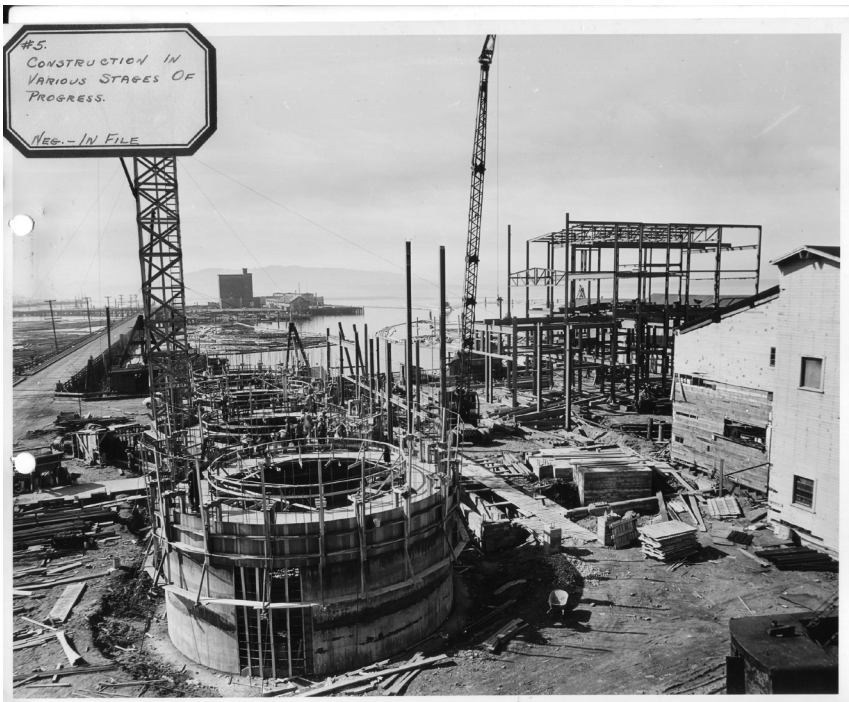
Pulp mill facilities. Source: Georgia Pacific.
