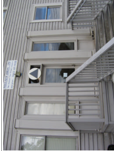
View of North front entry detail taken 8/29/2006
