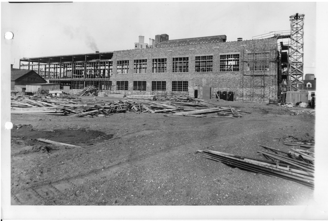
1947 view of construction of pulp mill facilities. Source: Georgia Pacific.
