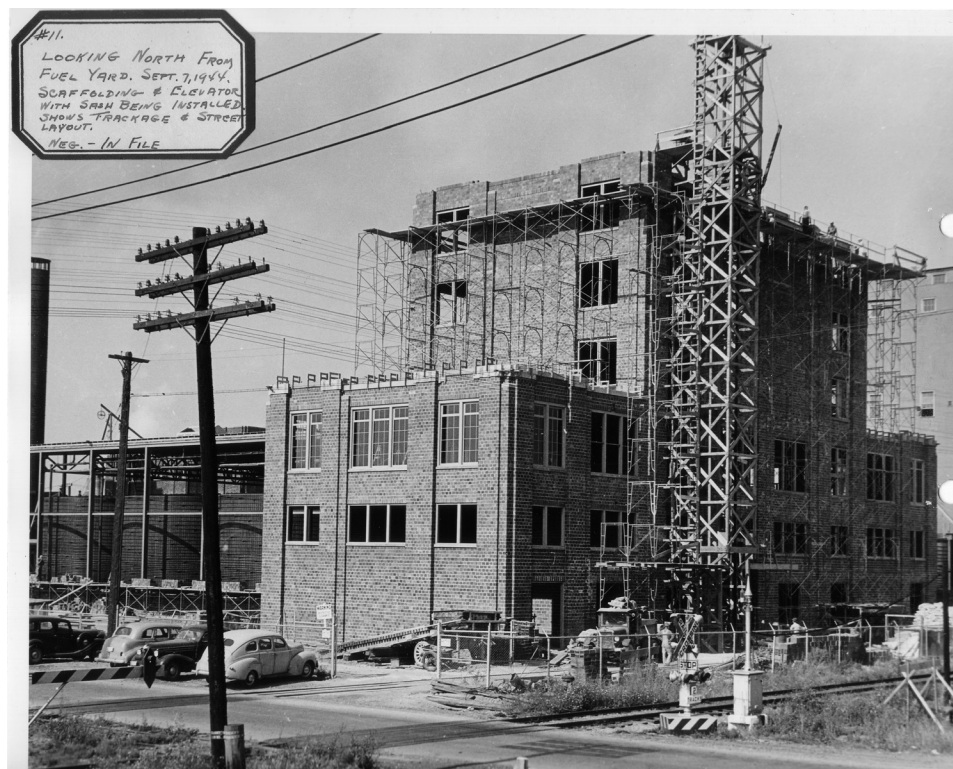
1944 view of construction of pulp mill facilities. Source: Georgia Pacific.
