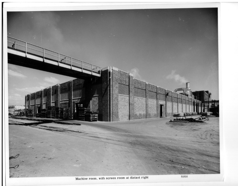
Pulp mill facilities. Source: Georgia Pacific.
